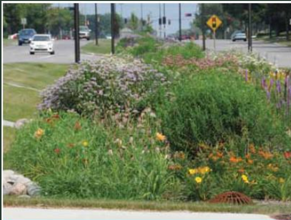
Bio-retention swales for stormwater treatment along Grange Avenue in the Village of Greendale.
