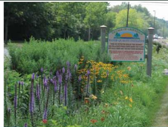
Bio-retention swales for stormwater treatment along Grange Avenue in the Village of Greendale.
