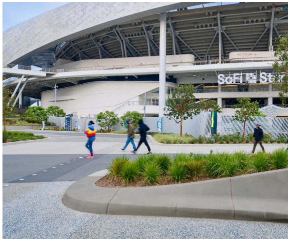
SoFi Stadium, California, HKS architects and MLA studio
