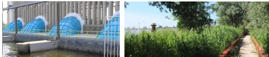
Pumping stations + green embankments
