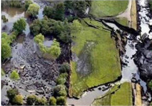
Levee subsidence (drought)
